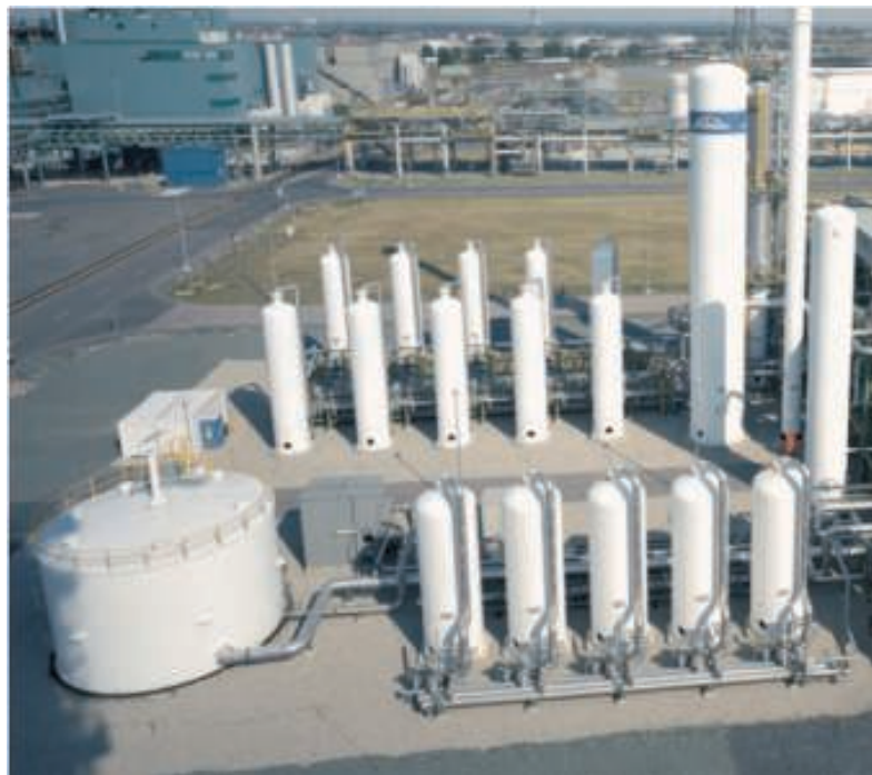
FIGURE 5. The plant scene depicted here shows a system for recovering CO 2 from the tailgas of a H 2 PSA system
