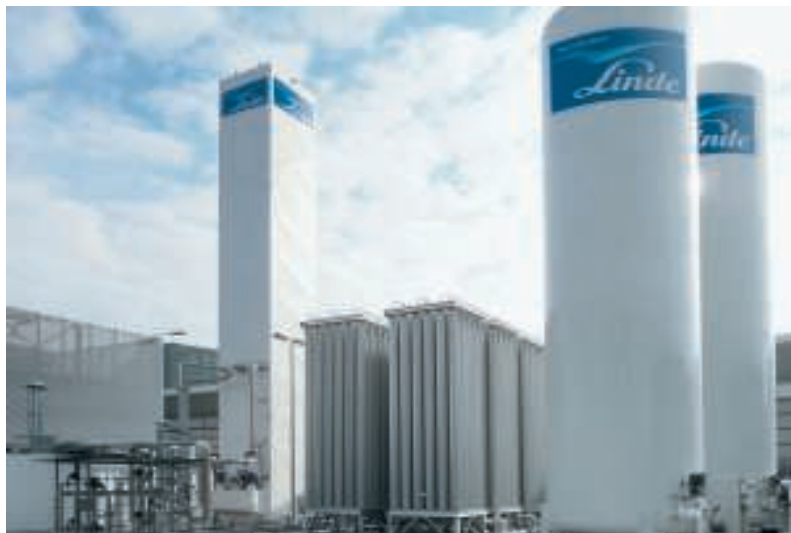
FIGURE 4. Modular gas plants, such as this Ecovar plant, are installed around the world for the dedicated production of oxygen, nitrogen, hydrogen or other industrial gases. Linde owns and operates the plants, monitoring and controlling production remotely. They deliver reliable, low-cost supply with no upfront investment cost, no overhead costs for labor, and no operating risk
